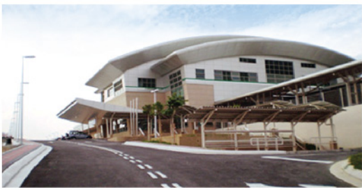
Electrified Double Track Project From Ipoh To Padang Besar
